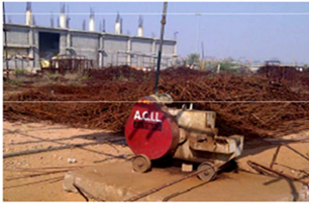
Fig. 6. Huge wastage of rebar by semi automatic machines [1]
