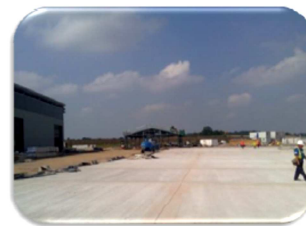
Hard Faced Storage Yard
