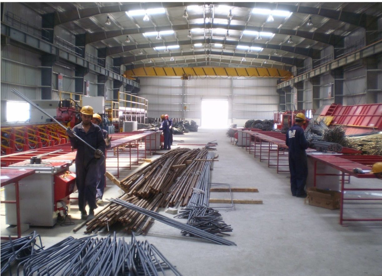
Fig.14 CBBY in operation at SUMPP (Inside view)
