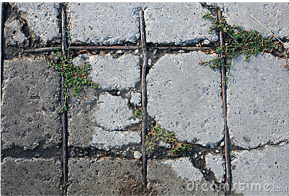
Fig. 7. Rusting/ mudding of rebars form weak bond with concrete.
