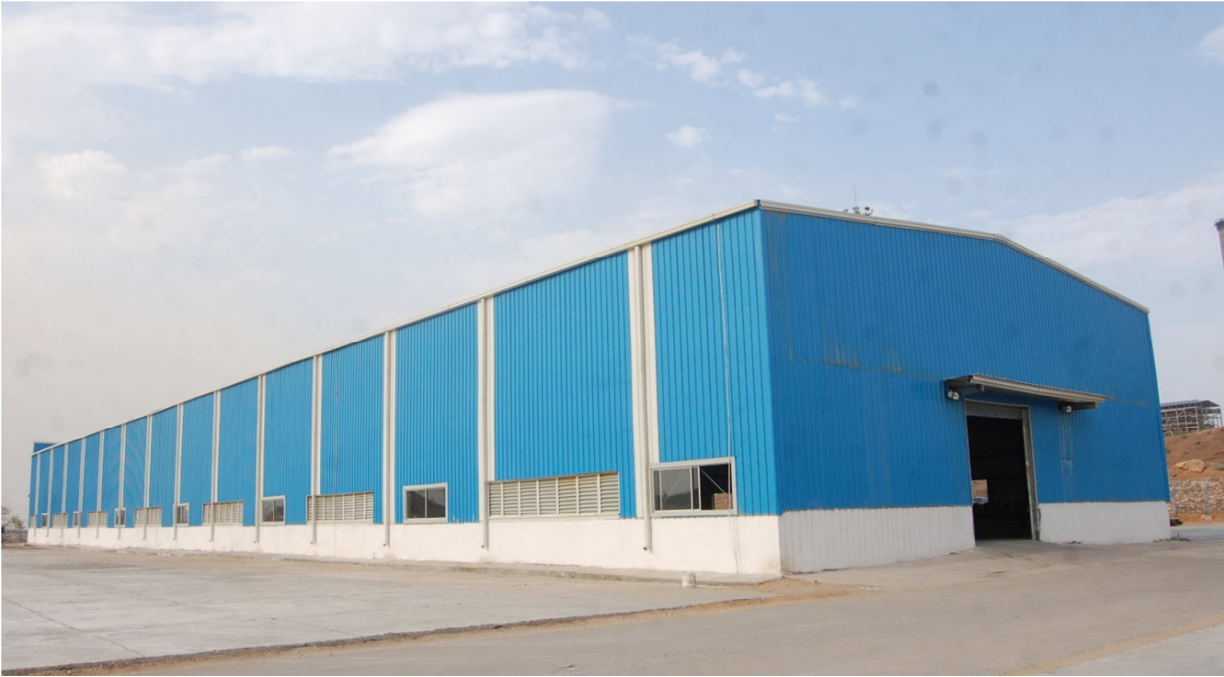
Fig.13 CBBY shed at Sasan UMPP outside view
